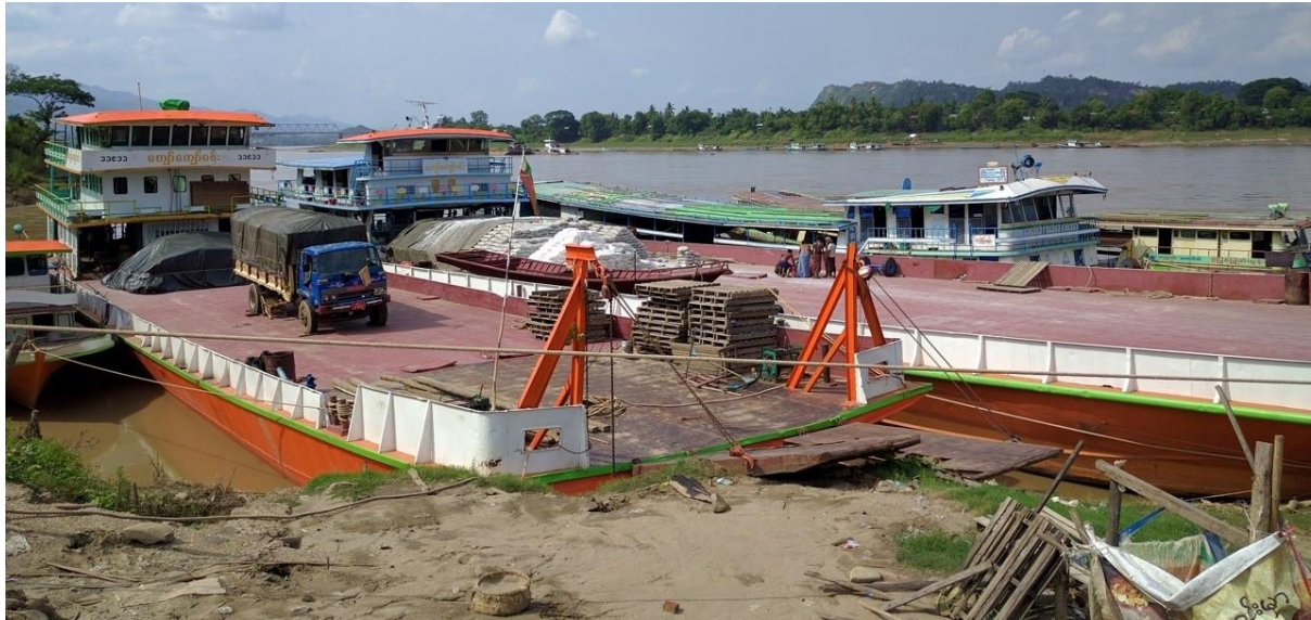
Figure 2 Kalewa Cargo port (Photo: LCA)
